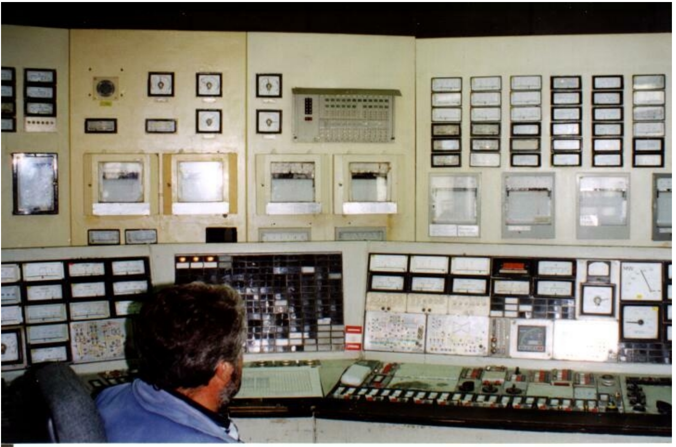
Figure 5a. Base shield for control 1 before the reconstruction
