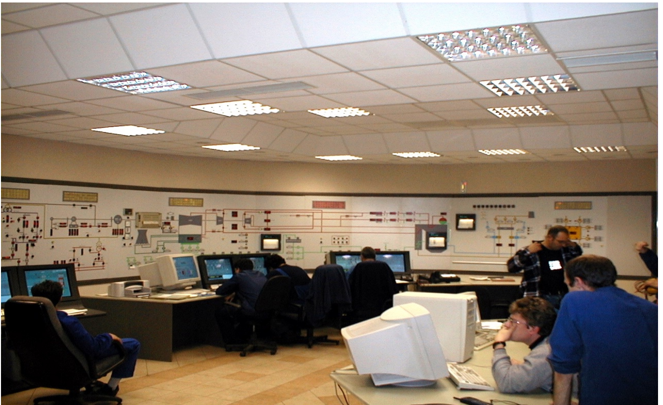
Figure 5b. Base shield for control 1 after the reconstruction
